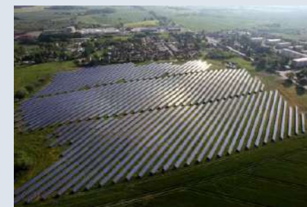
4.8 MWp PV plant in Bobitz (Germany)
