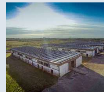
220 kWp PV-Anlage in Petrovija (Croatia)
